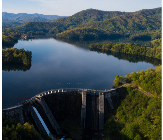
Santeetlah hydropower facility (Source: Brookfield Renewable U.S.)
